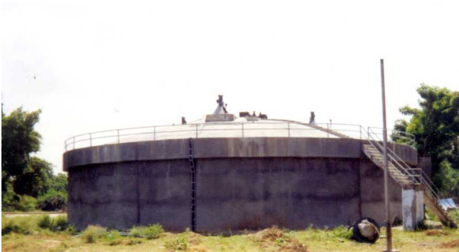
Anaerobic Digester Tanks with Multiple Draft-Tube Digester Mixers
