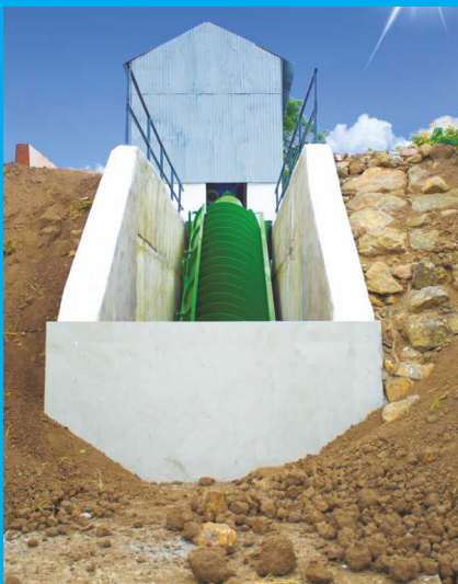
18.5kW Hydropower station at IMC, Indore
