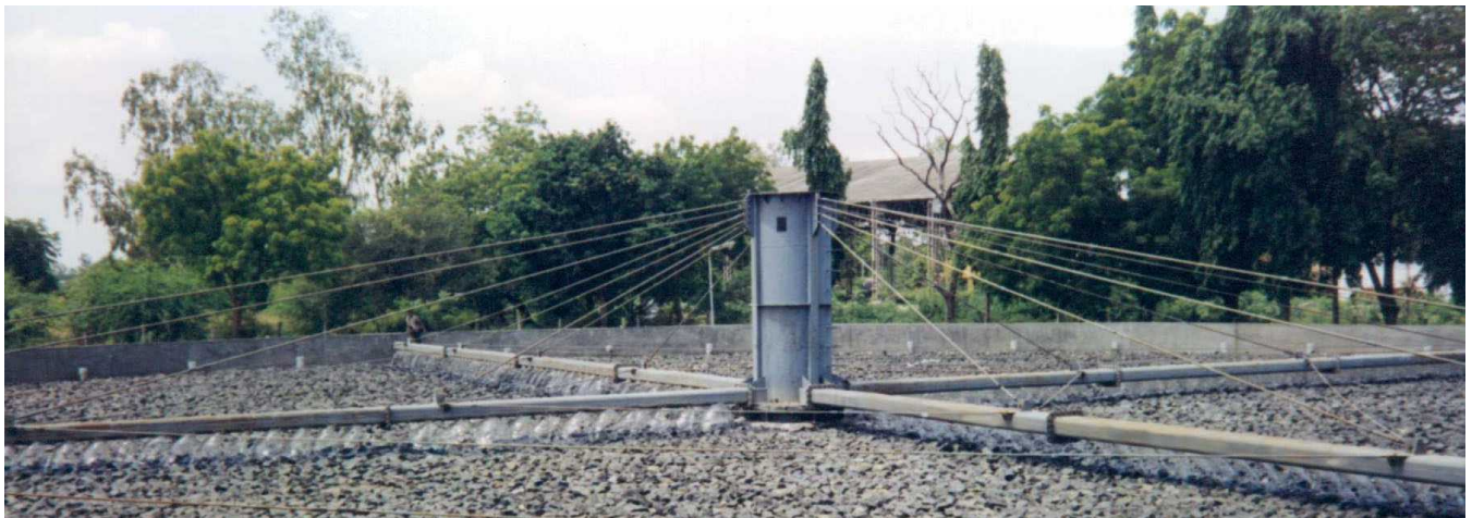
48m dia Trickling Filter at Atladra STP – Baroda
