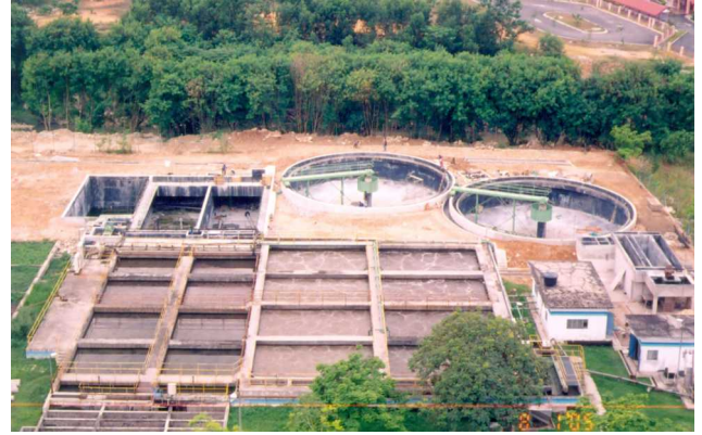
STP at Damansara, West Malaysia
