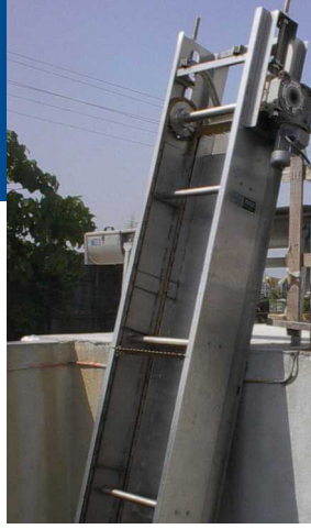
Type SP-M2-C Mechanical Coarse Screen Installation at Kimdec, Malaysia
