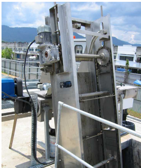
Type SP-M2-C Mechanical Fine Screen Taman Mas, Sewage Treatment Plant, Malaysia
